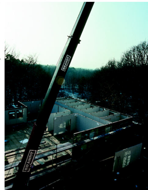
Construction of PIK's provisional building on the Telegrafenberg in Potsdam.
