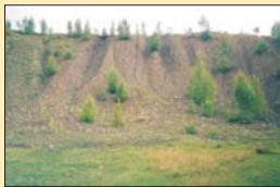
Waste slopes affected by gully erosion. In rare cases, some species, like Betula nana , appear spontaneously on the slopes
