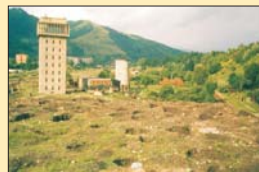
Compaction on waste dumps at Petritu
